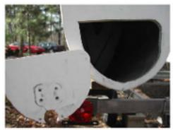
Cut the transom section out with a coarse-bladed reciprocating saw. Save the piece to put it back in later. Be careful to retain the steel plate in its original location, so the gudgeon screws will line up again.
